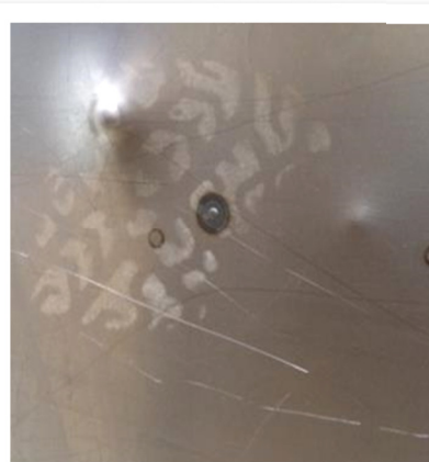
Door interior-shots do not penetrate
